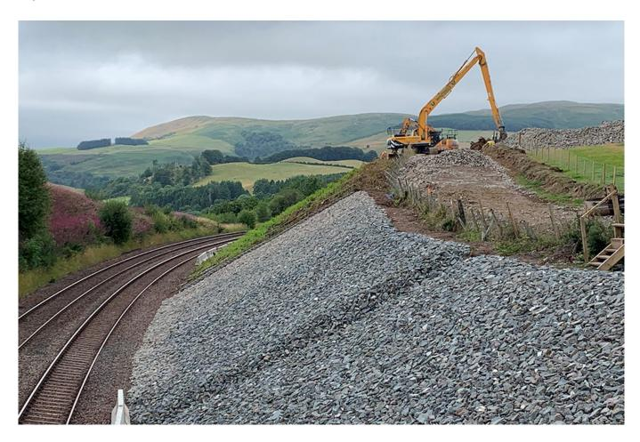
Work is underway to upgrade drainage systems and re-profile embankments to reduce the risk of flooding and landslips on the line between Sanquhar and Dumfries.
