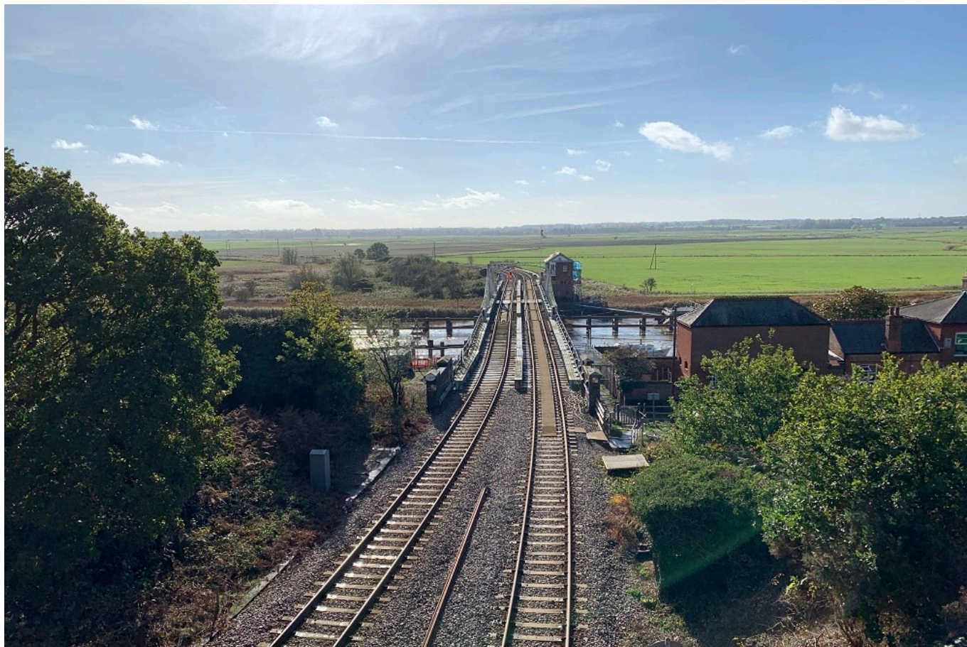
View of Reedham swing bridge
