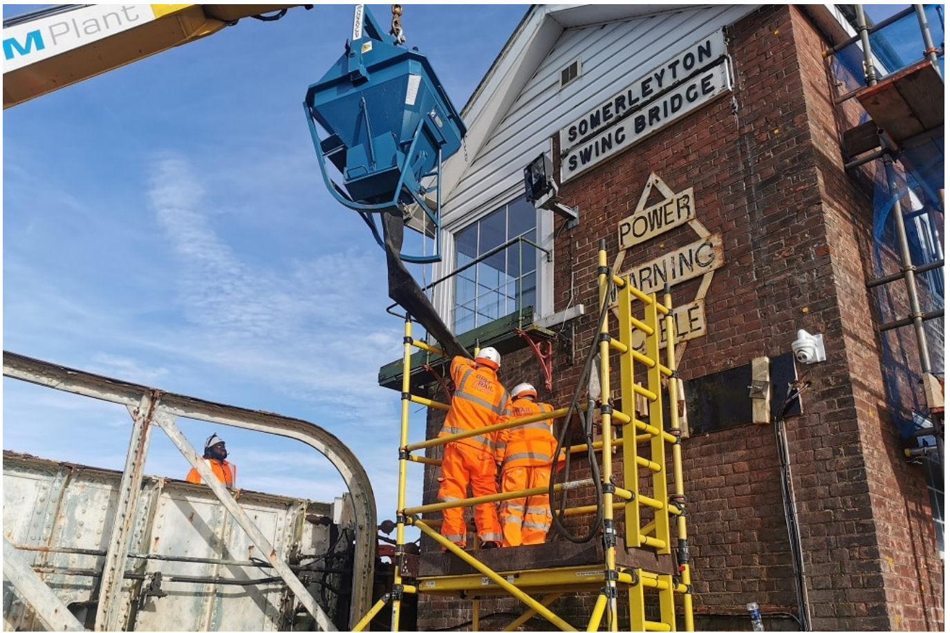
Beam installation at Somerleyton swing bridge
