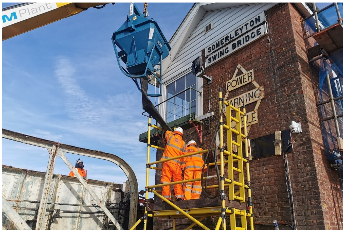
Beam installation at Somerleyton swing bridge
