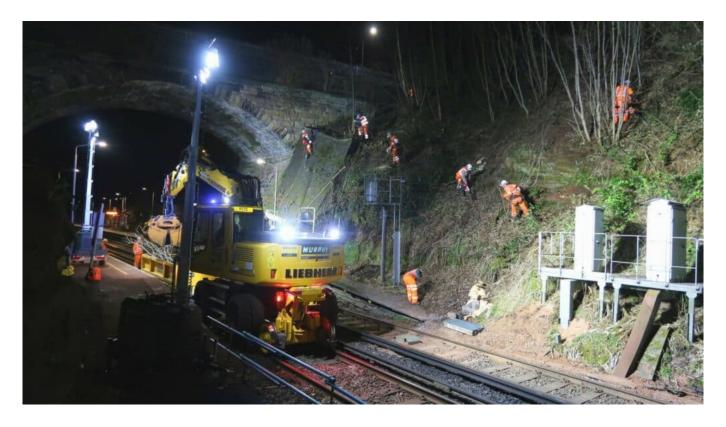
Abseiling teams have been securing a steep railway cutting making it more reliable for passengers on the line between Liverpool and Ormskirk.
