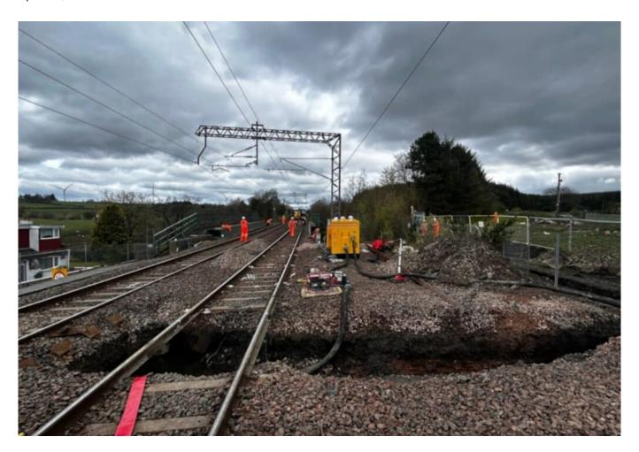
The line between Airdrie and Bathgate is expected to remain closed until Monday 29 April, due to the potentially complex nature of the repairs needed to the railway. It comes after a sinkhole was discovered by track engineers on 21 April with the line being closed to allow investigation work to be undertaken.
