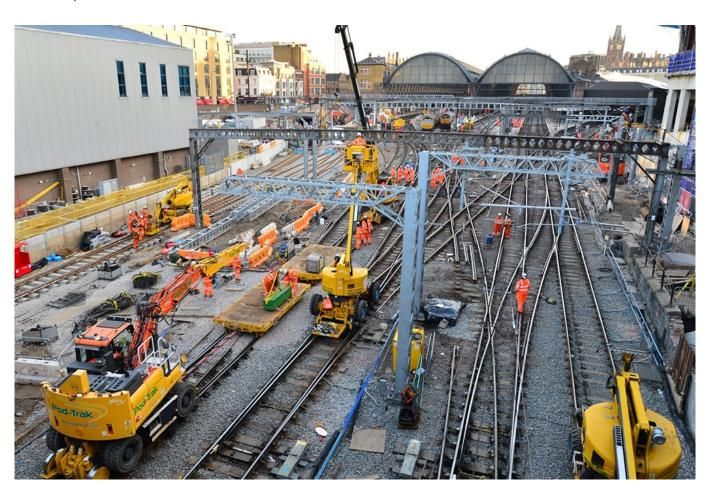
Platform edges have been demolished, track has been lifted and overhead line equipment has been removed as London King's Cross prepares for its biggest platform alteration next month.
