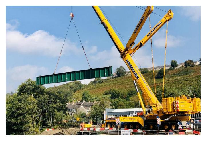
At 06:30 on Monday 28th September AmcoGiffen and Network Rail successfully re-opened the River Ebbw Bridge on schedule to rail traffic following an intensive programme of replacing and increasing the capacity of the time-expired structure.
