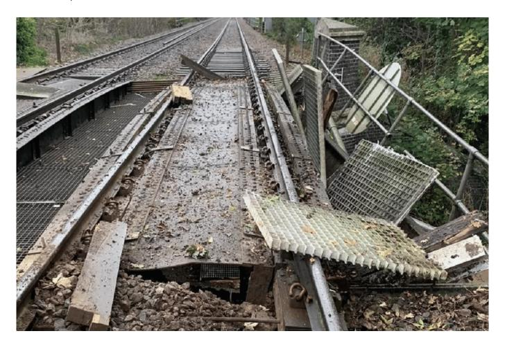
Significant damage has been caused to a bridge at Ketton, between Leicester and Peterborough after it was struck by a lorry on Saturday, 5 November. Critical parts of the bridge structure have been so badly damaged that a significant part of it needs to be replaced.
