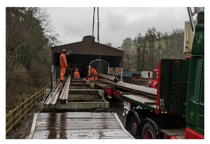
British Steel's ongoing support for UK heritage railways has continued with a sizeable delivery of brand new, 95 pound/ metre, or 47.07 kg / metre, bullhead rail to the South Devon Railway (SDR) which was rolled at British Steel Scunthorpe.
