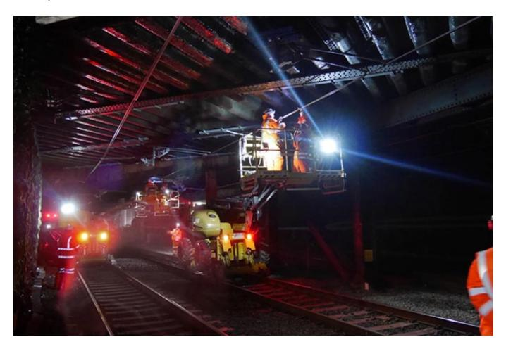
In a world first, electric resistant paint combined with voltage-controlled clearance (VCC) has helped make a Victorian railway bridge usable by new electric trains, avoiding weeks of passenger disruption and train delays in the process.
