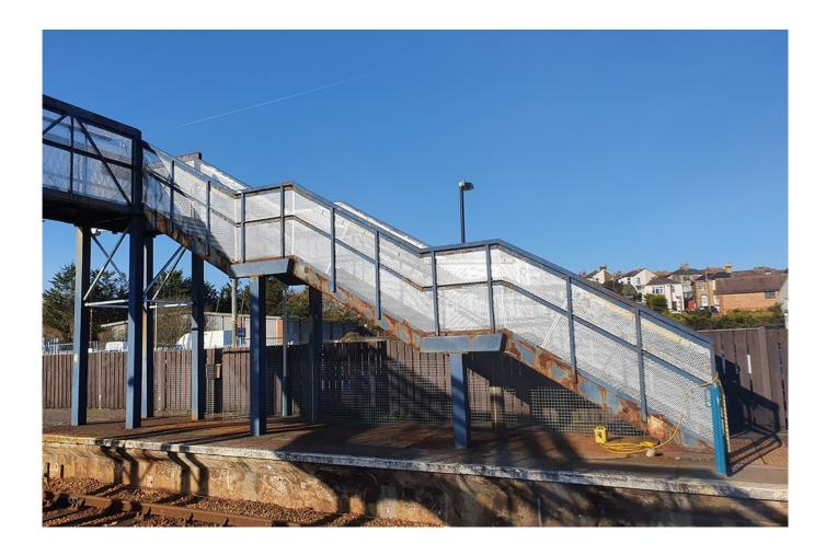
A similarly satisfying project that we also completed whilst the country was in lockdown is Bookham Station structure refurbishment. Again, the metallic structure was prepared by our teams to St3 sound surface standard and a protective paint system was applied with all works being carried out during dedicated night time closures. Check out our project case study here:
