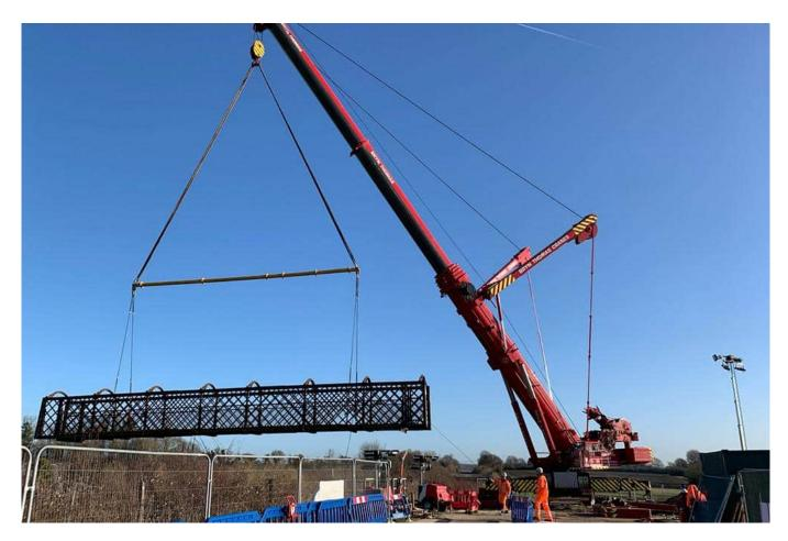
Dyer & Butler, a multi-disciplined engineering services specialist focused on essential infrastructure including airports, railways and highways, and part of M Group Services, has completed the replacement and installation of a new footbridge spanning two electrified (third rail) running lines at Cobham.
