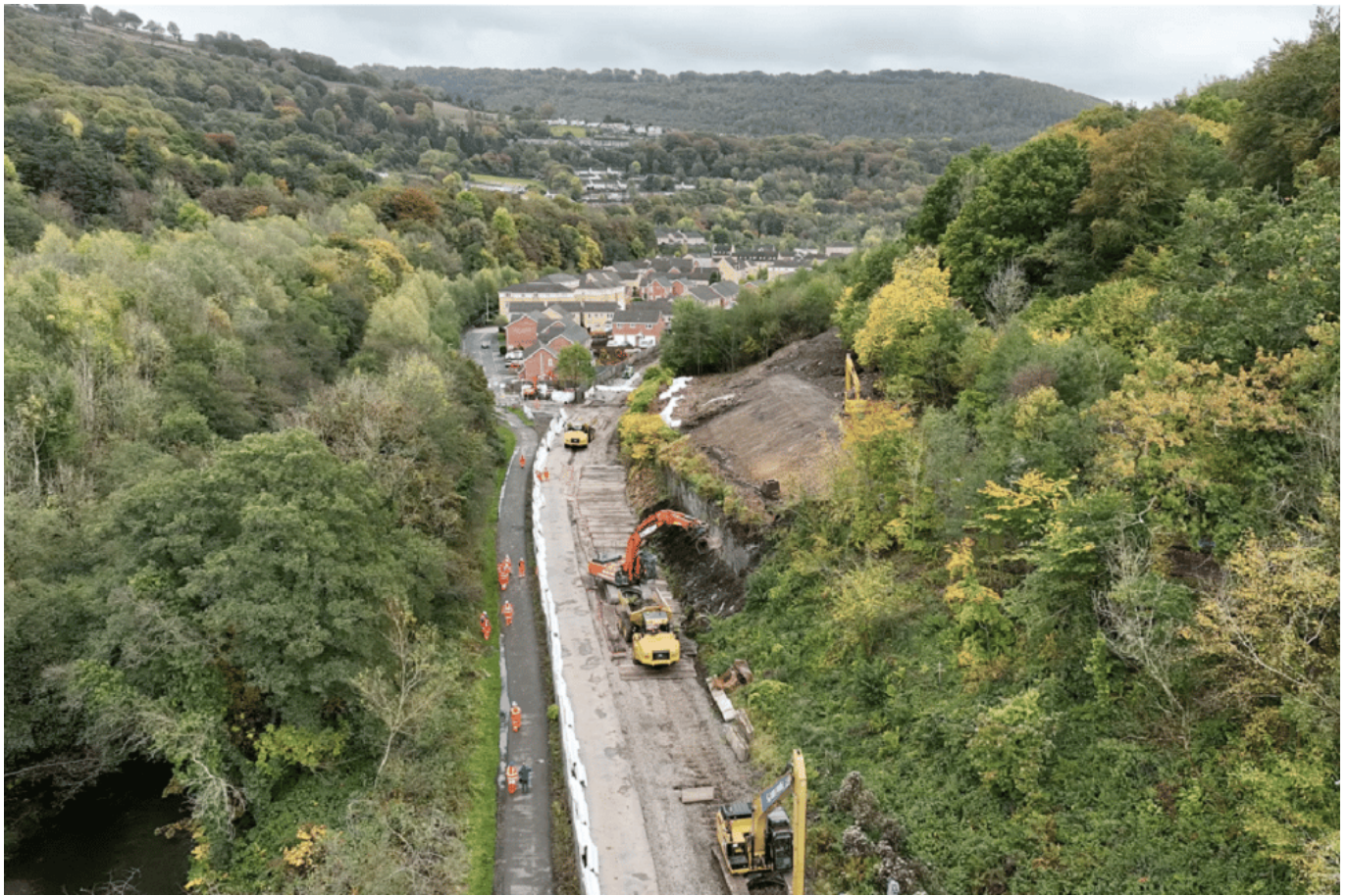
Removal of the retaining wall
