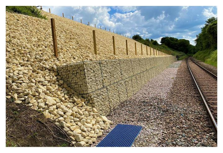
Essential work to reinforce the embankment and protect the tracks on the Sudbury branch line has been carried out to prevent delays and cancellations to the rail service.
