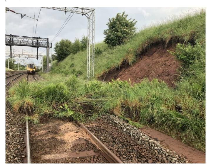
Emergency landslip repairs have been made after 180 tonnes of earth slipped onto the railway after persistent heavy rainfall near Whitmore, Staffordshire.
