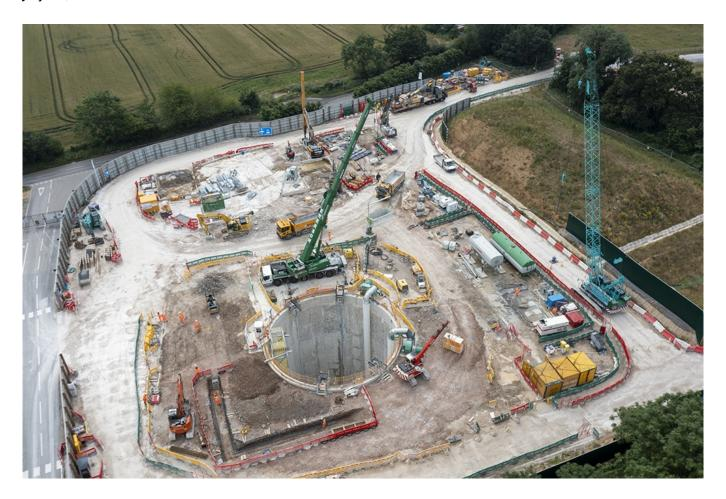
Following the launch of the first two giant tunnelling machines at HS2's nearby South Portal site, engineers working on Britain's new high speed railway have now begun excavating the first of five shafts that will provide ventilation and emergency access to HS2's ten-mile long tunnels under the Chiltern hills.
