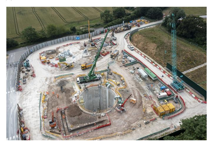
Following the launch of the first two giant tunnelling machines at HS2's nearby South Portal site, engineers working on Britain's new high speed railway have now begun excavating the first of five shafts that will provide ventilation and emergency access to HS2's ten-mile long tunnels under the Chiltern hills.
