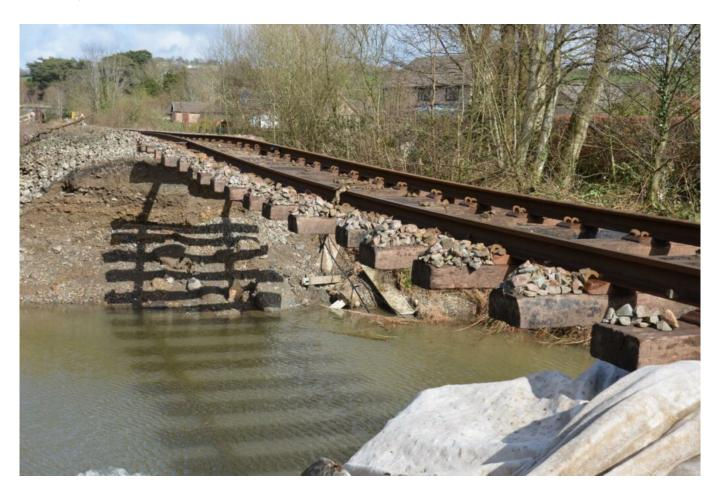
Drone footage released by Network Rail Wales and Borders shows the extensive damage caused by Storm Gareth on the Conwy Valley Line. The line, which runs between Llandudno Junction and Blaenau Ffestniog, will remain closed for a number of months.
