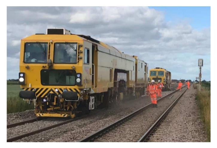
Track, sleepers and ballast have been replaced by Network Rail's engineers as part of a programme of upgrade works to make train services more reliable between Ipswich, Ely and Cambridge.
