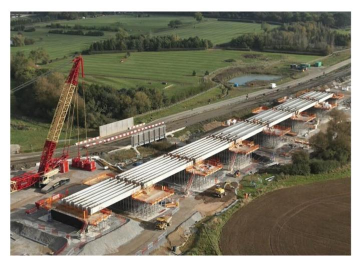
A viaduct in Northamptonshire has become the first on the HS2 project to have all its deck beams installed as work on the project continues to ramp up between London and the West Midlands.
