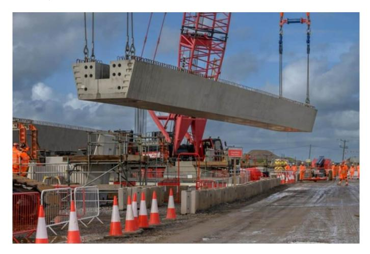
HS2 has begun lifting the first of 72 huge beams that will support the deck of the Thame Valley Viaduct – the first of its kind in the UK to have all major elements manufactured off site.
