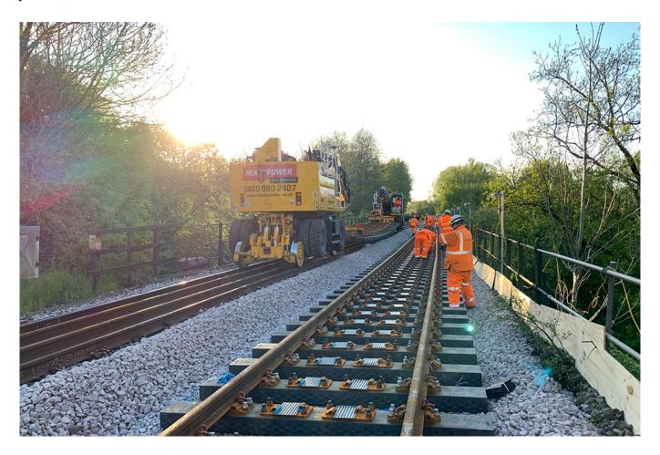
Trains in Wiltshire are now running on top of old bottles, food packaging and other unwanted plastics, with the introduction of the first composite railway sleepers on Network Rail's main line tracks.
