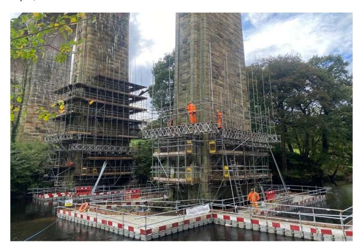
Floating Pontoon Solutions has supported AmcoGiffen's refurbishment of the Cefn Viaduct in Merthyr Tydfil, Wales to allow brickwork repairs to take place on the historic structure.
