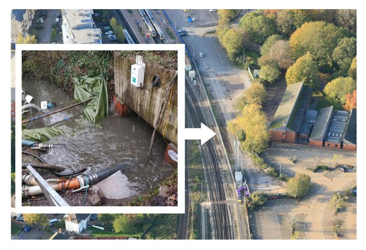
Network Rail engineers are carrying out emergency repairs to a damaged culvert which takes a waterway under tracks to the south of Aylesbury station.
