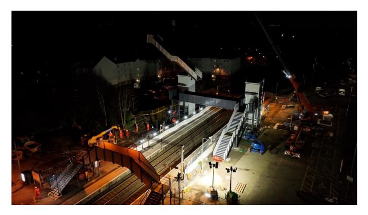
A new fully accessible footbridge and lift towers have been installed at Uddingston station.
