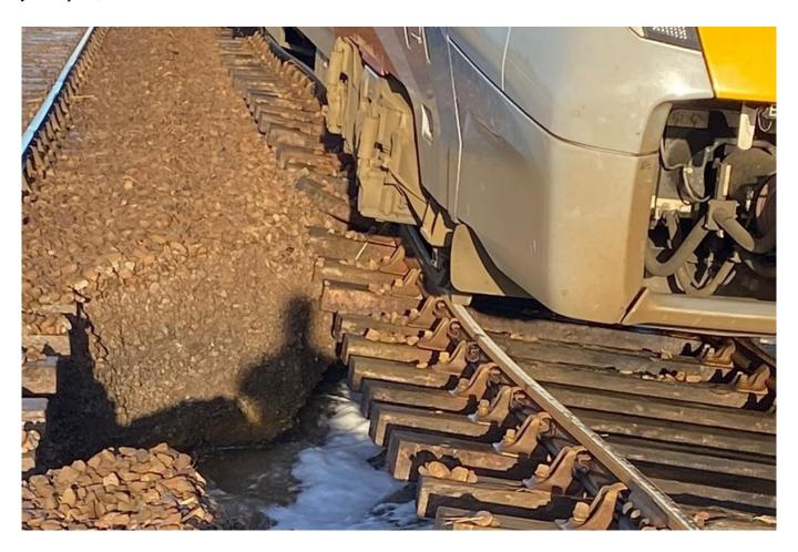
Rail passengers were led to safety after a very high tide and winds caused ballast, to be washed away at Haddiscoe on the Norwich to Lowestoft line.
