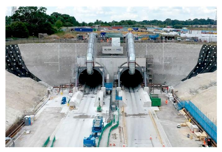
Two enormous 2,000 tonne tunnel boring machines (TBMs) digging HS2's longest tunnels passed the second of five ventilation shafts this week, four miles into their 10 mile drive under the Chilterns.
