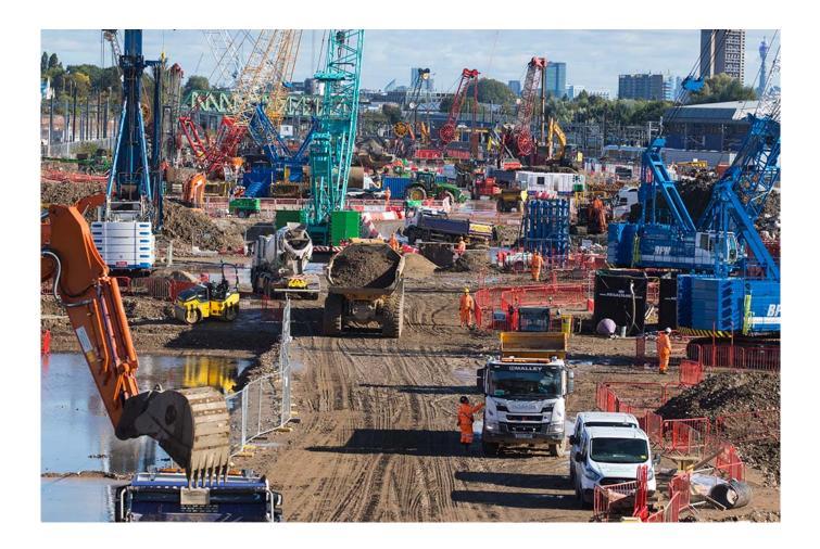
Expanded – part of Laing O'Rourke – will excavate 20m below ground level removing 690,000 cubic metres of clay, before placing 32,000 tonnes of steel and pouring 190,000 cubic tonnes of reinforced concrete. This type of excavation, known as "top down" construction, allows the ground floor slab to be made initially with a series of "mole holes" allowing access for the large excavators to remove the earth from within.
