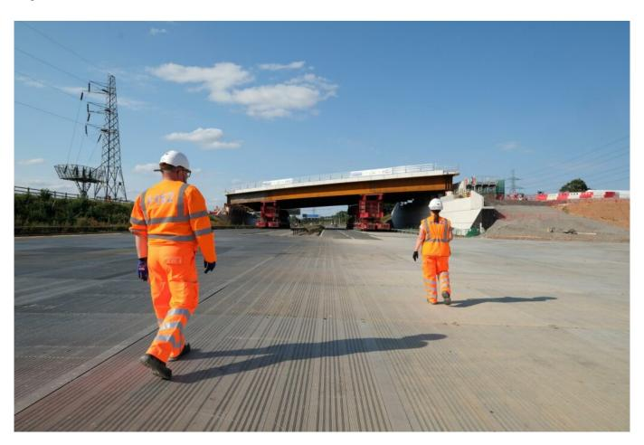
Work to install a 65-metre bridge, spanning the width of the M42, was completed in just two days and ahead of schedule as the motorway reopened to road users on Sunday (9th August) 22 hours earlier than planned. The works near Interchange Station move Solihull a step closer to the arrival of HS2, Britain's new low carbon high speed railway.
