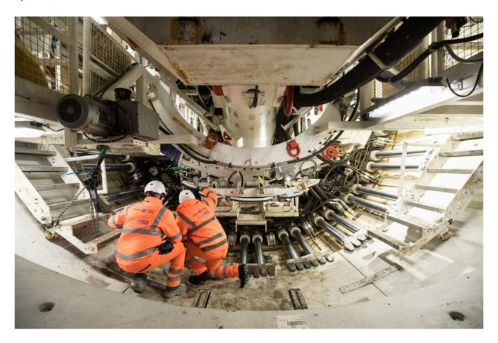
HS2 has once again begun tunnelling under the capital, launching its third giant Tunnel Boring Machine (TBM) in London. The tunnel won't be used by HS2 trains, but instead will be used to deliver materials and remove spoil from the northern portal where HS2's Euston twin bored Tunnel will be constructed.
