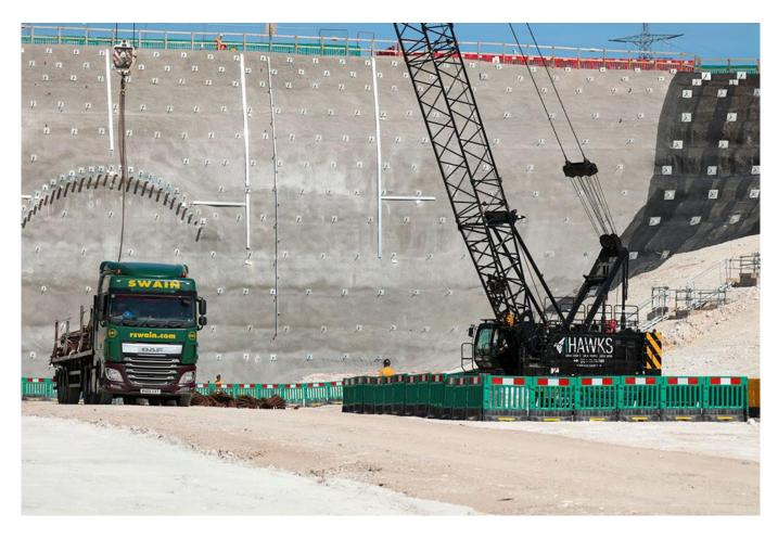
Preparation for the arrival of HS2's first giant tunnelling machines has passed a major milestone with the completion of the 17m high headwall and ground reinforcement at what will become the south portal of the 10-mile long Chiltern tunnel.
