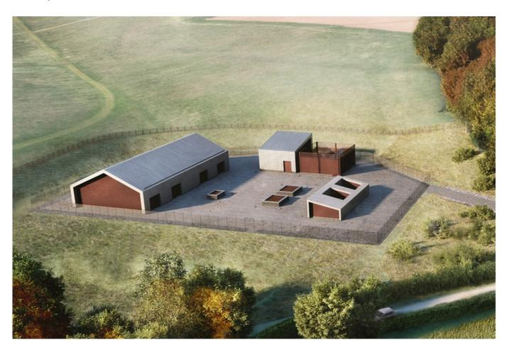
HS2 has revealed the final design for the latest of its 'barn design' headhouses that will provide ventilation and emergency access to the ten-mile long Chiltern tunnel.
