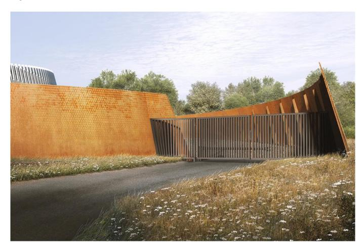
HS2 has revealed the design for the Amersham vent shaft headhouse – one of five structures that will be built to provide ventilation and emergency access to the high-speed rail line's 10 mile-long Chiltern tunnel.
