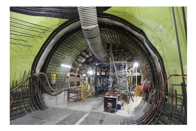
The work to construct the tunnel took 16 months and saw the MDJV team sink a 20-metre deep shaft before carving out the underground passage and coating it with a primary sprayed concrete lining (SCL). After applying waterproofing, the team reinforced the tunnel with steel and concrete to give it the strength and structure needed ahead of the construction of the HS2 Station that will be taking place above it.
