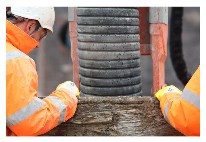
HS2 Ltd has revealed a new vacuum excavation technique for piling which could have massive benefits for the wider construction industry in the UK and abroad. The innovation, developed by specialist contractors working on HS2, is better for the environment, safer for workers and reduces construction noise, to the benefit of neighbouring communities and businesses.
