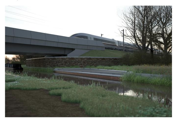
HS2 says that traditional Warwickshire 'ironstone' will be used to clad the piers supporting the high speed railway's new Oxford Canal Viaduct as a nod to the canal's architectural heritage after engaging with the local community.
