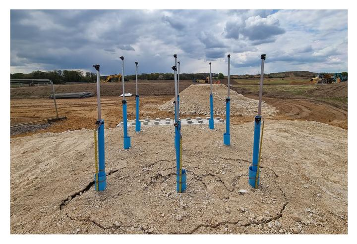
An HS2 construction site is the test bed for a potentially far-reaching fibre optic technology that can sense minute ground movements in embankments and cuttings, and could help prevent land slips and detect the formation of sink holes.
