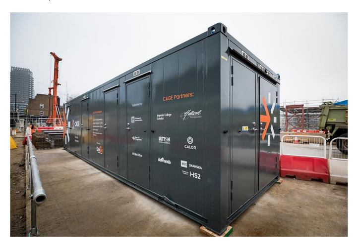
In its bid to cut carbon and focus on improving local air quality, HS2 is trialing new ultra-clean generator technology developed by a collaboration of three UK technology companies. By replacing diesel with LPG, the innovation is set to cut carbon, lower emissions, reduce noise and deliver major cost savings.
