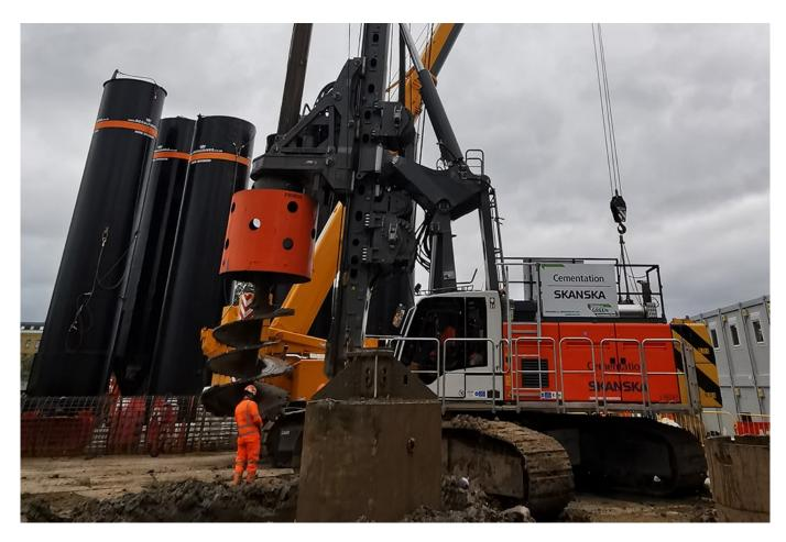
HS2 has announced a pioneering project to use Hydro-treated Vegetable Oil (HVO) for the first time in the UK in a piling rig on an HS2 site in London, the largest engine ever to trial its use. HS2's contractor Skanska Costain STRABAG joint venture (SCS JV), through Cementation Skanska, has been undertaking a three-week trial to find more eco-friendly fuels to use on construction sites for piling activities.
