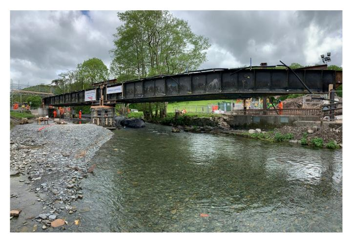
Network Rail engineers are working through extreme weather to raise Black Bridge, near Machynlleth, by one metre to lift it out of the flood zone.
