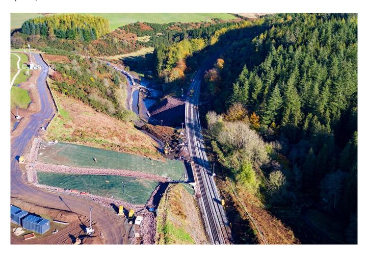
An interim report by the Rail Accident Investigation Branch (RAIB) into the Stonehaven tragedy has revealed the train derailed after colliding with stones washed out onto the track from the gravel-filled crest drain and from the adjacent ground.
