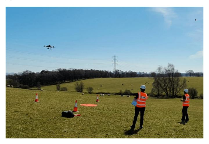
Keltbray, a leading specialist engineering business and provider of overhead line and substation services, is using drones to double inspection efficiency and cut carbon emissions by almost 50 per cent.
