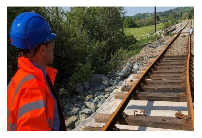
The damage to the railway which was caused by a combination of high tide and a low pressure system following storm Gareth in March has affected 6 miles of track.
