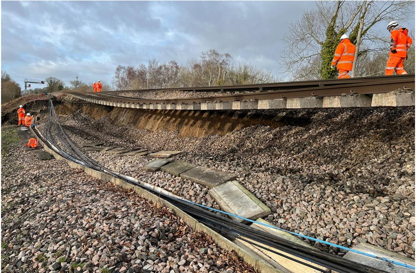
A large landslip in Hampshire has left one of the tracks of the main line from London to Basingstoke hanging in mid-air, one other track damaged, and huge disruption expected for customers.
