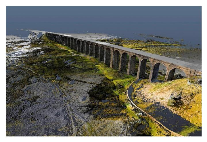
Laser scanners and drones have been used to map every inch of the iconic Ribblehead viaduct as part of a major restoration project to secure its future for passengers and tourists.
