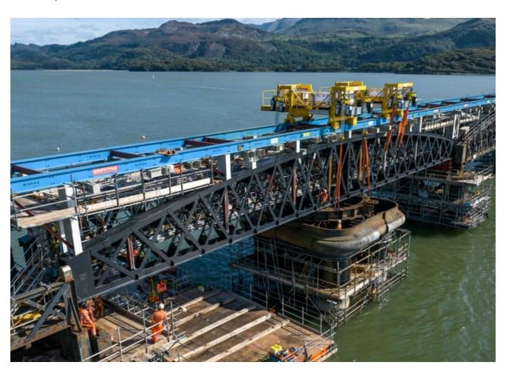
Network Rail has successfully moved two new 160-tonne metallic spans into place onto Barmouth Viaduct, reaching a milestone in the restoration of the iconic structure.
