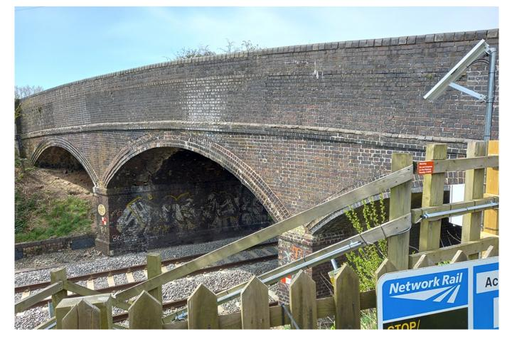
A bridge in Great Glen, Leicestershire, is being raised by Network Rail, to clear the way for train-powering electric wires to be installed in the future.
