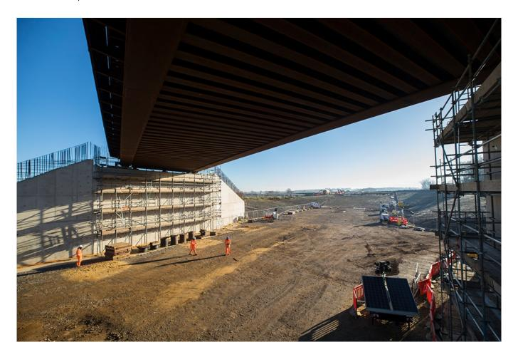
A new bridge that will carry direct rail services between Oxford and Cambridge has been lifted into position over the route of HS2, the high speed rail line under construction between London, Birmingham and the North.
