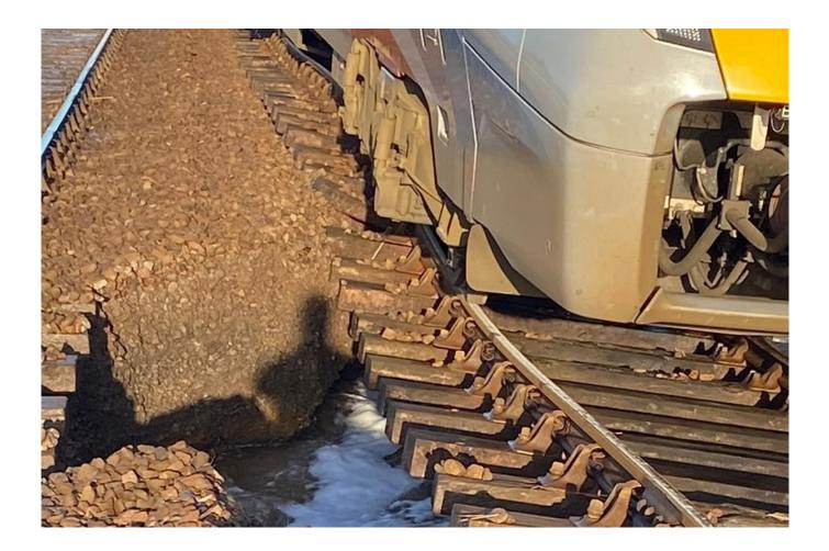
Up to 500 tonnes of rock and ballast have been used to reinstate the embankment under the track bed to replace the original material that was washed away.
