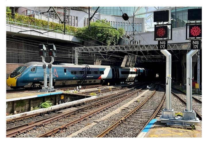
Birmingham New Street station signalling system has gone digital. Over the last 15 months more than 230 miles of cabling has been laid to connect 64 new LED colour light signals at Birmingham New Street station.
