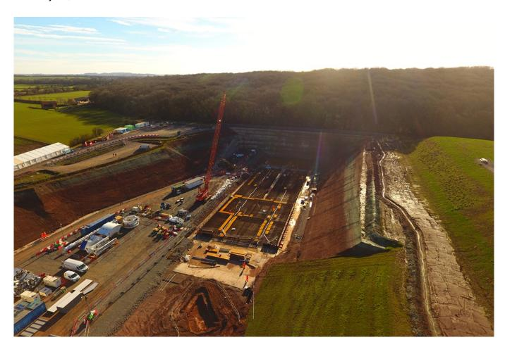
Midlands-based construction firm, Collins Earthworks, has completed excavating the north portal site of Long Itchington Wood Tunnel, ready for the launch of the tunnel boring machine that will dig under the ancient woodland in Warwickshire.
